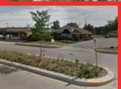
Instead of proper bioretention - these convex impervious areas do not capture water & utilize the runoff, they
